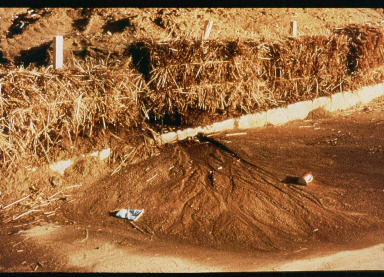
Typical straw bale installation (failure)
