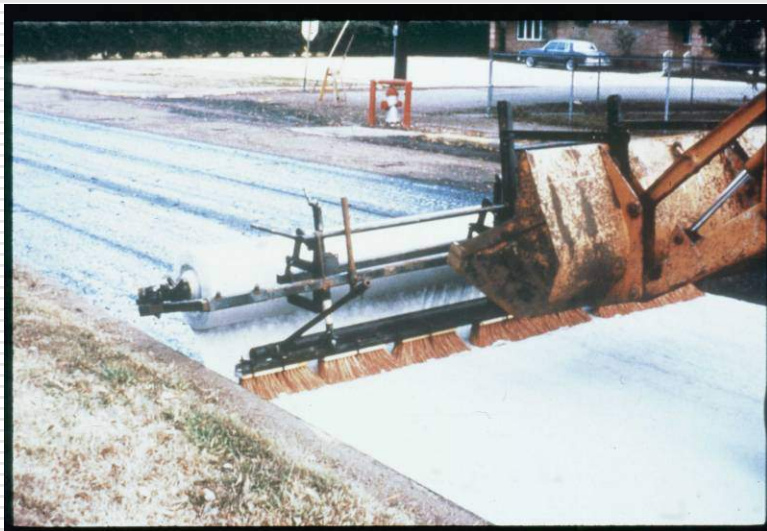
Paving Fabric for Overlay Stress Absorption & Waterproofing
