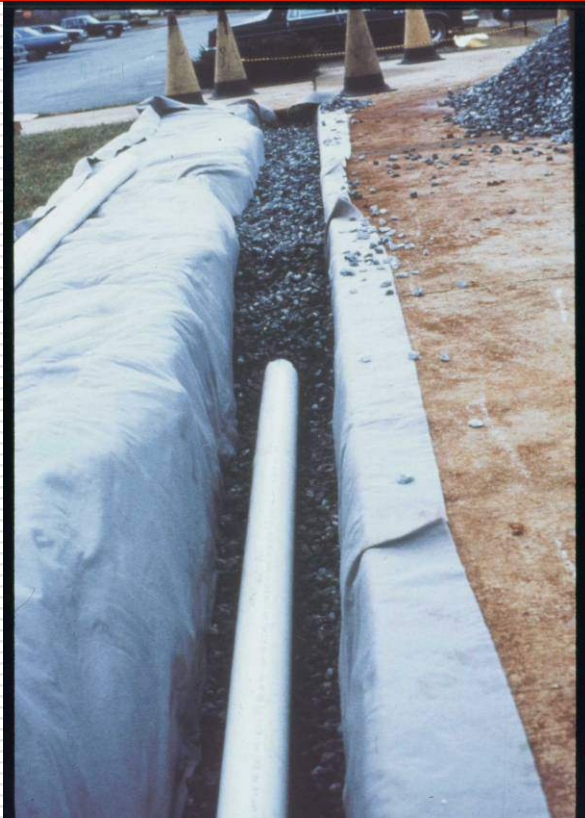
Placement of coarse aggregate and pipe.
