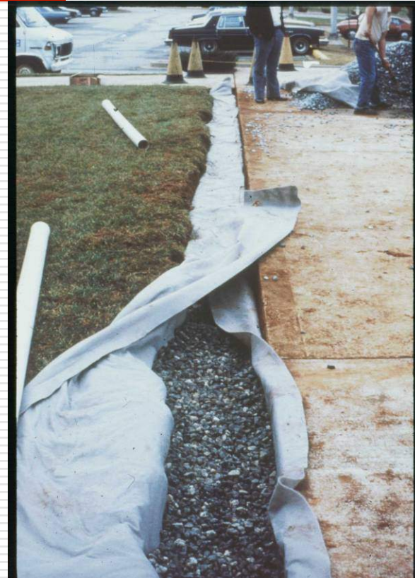
Completion of drain by wrapping the geotextile. Then backfill to grade.
