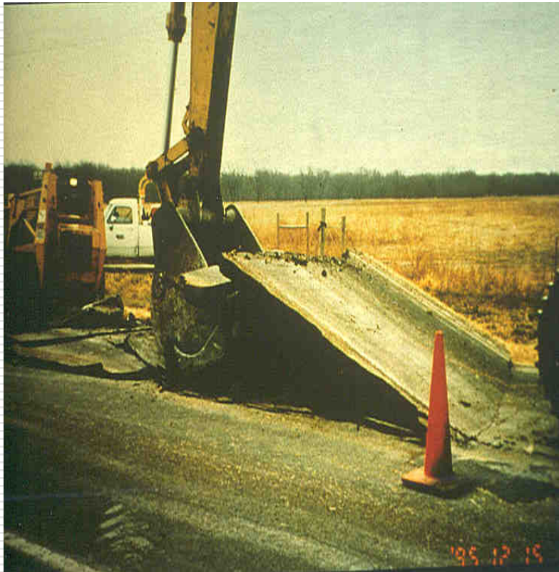
Remove Fouled Sections
