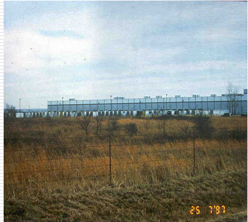
New Appliance Factory
