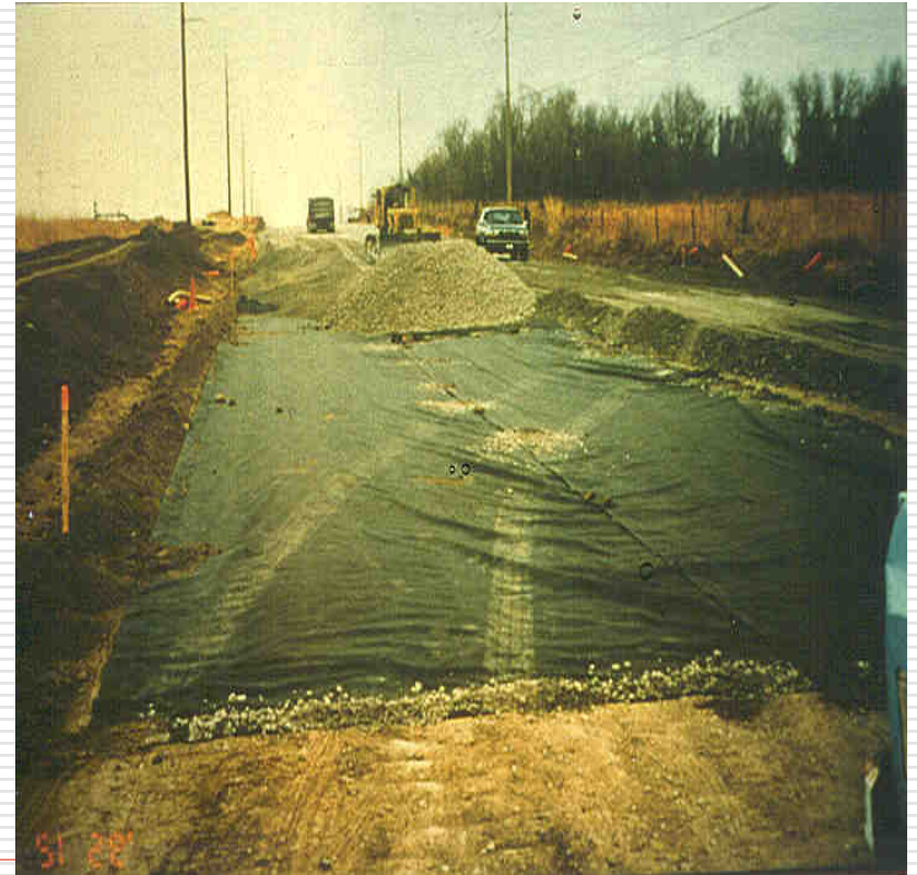
Install Separator
