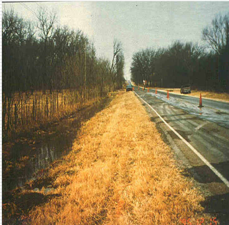
Existing Rural Road
