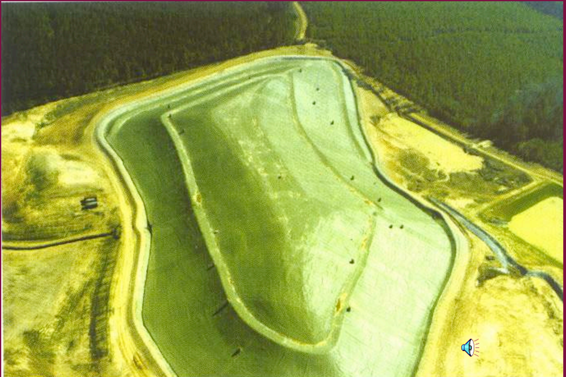
A 16-acre EGMC placed over MSW landfill in Louisiana.
