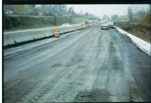
Geogrid base reinforcement stiffens the aggregate base layer providing long-term support for the paved surface.
