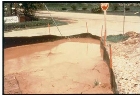
Silt fence retaining sediment laden runoff.
