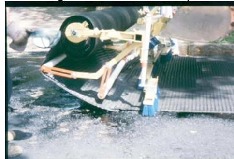
Paving Grid for Overlay Reinforcement
