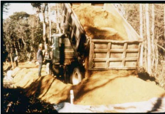
When constructing over weak subgrades, back-dumping of the aggregate is required
