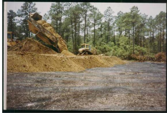
A geogrid is effective in reducing the required fill over a weak subgrade
