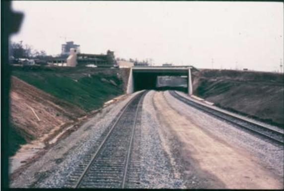
A new rail line in an area of high groundwater is built over a heavy weight nonwoven geotextile
