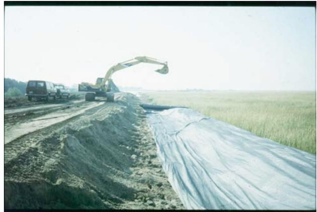
The fill thickness tapers toward the embankment toe to reduce the reinforcement requirements and allowing a lighter-weight geotextile to be used under the embankment slopes.
