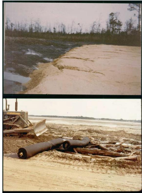
When more challenging subgrades are encountered it is usually more effective to leave vegetation and construction debris in place
