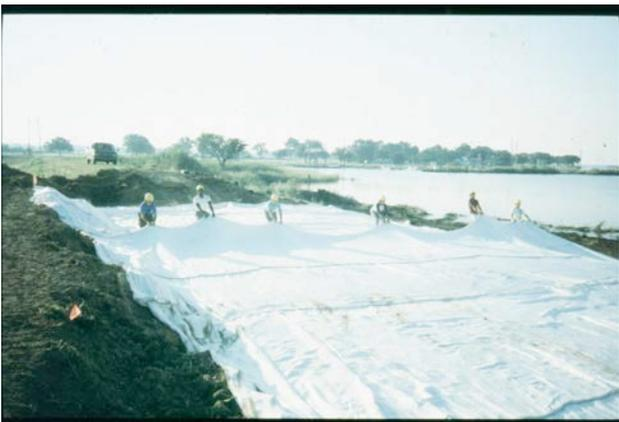
The connected panels are then positioned to assure that the reinforcement is oriented to maintain embankment stability.
