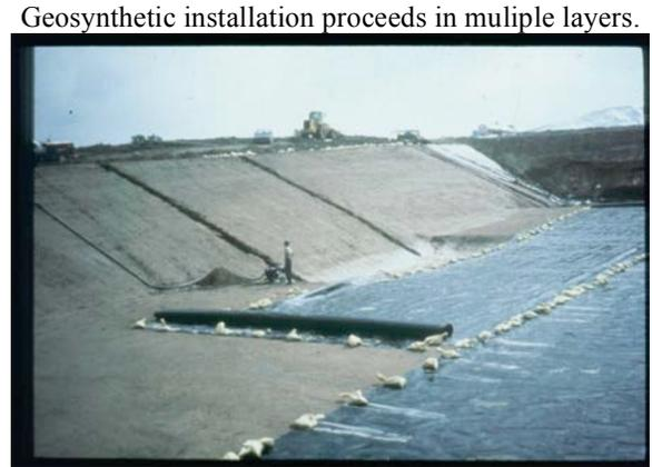
Geosynthetic installation proceeds in multiple layers.
