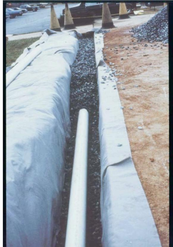
Placement of coarse aggregate and pipe
