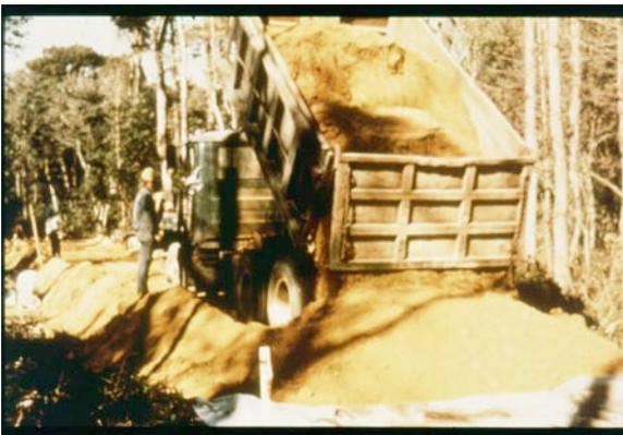
A stabilization geotextile facilitates construction over weak subgrades
