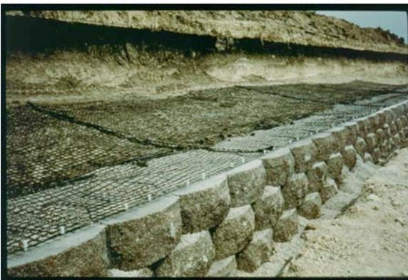
MSE walls have geosynthetic reinforcement layers.
