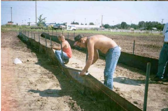
Silt fence installed in trench, backfilled and compacted; posts installed, and fabric tied to posts.
