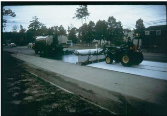
Tack Coat Application and Fabric Laydown
