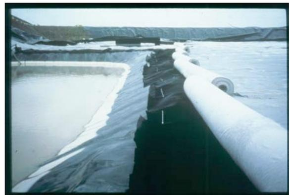
The leachate collection system drains to a lined sump.
