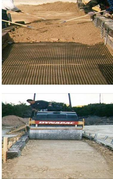
Installation damage testing determines how much the tensile strength of a product should be reduced to account for damage during construction
