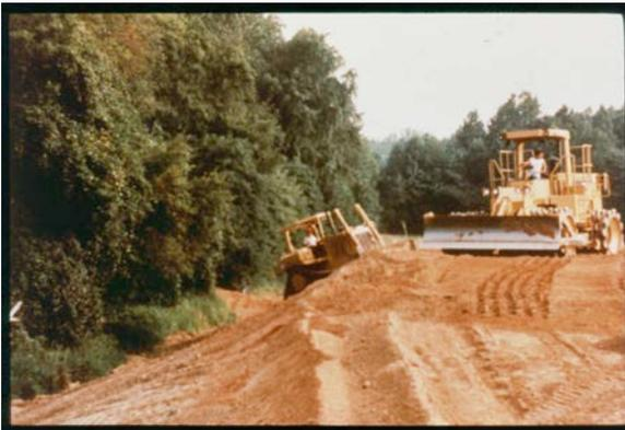
Alternating layers of geosynthetic and compacted soil.
