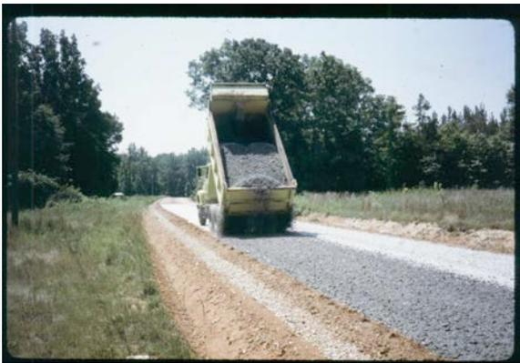
If the subgrade is firm and free of debris, run and dump placement of aggregate may be used
