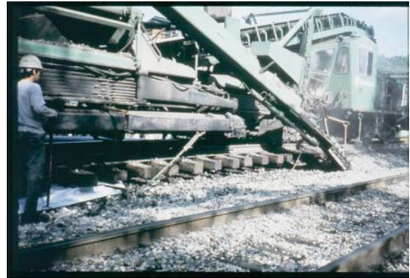
Railroad maintenance operations can include the insertion of a geotextile during undercutting
