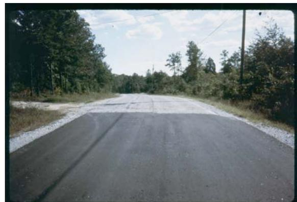
A surface treatment such as an asphalt layer or a double or triple-treatment can be placed once the base course is complete and structurally sound.
