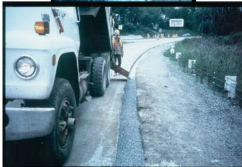
The trench is "lined" with the filtration geotextile prior to pipe and aggregate placement.
