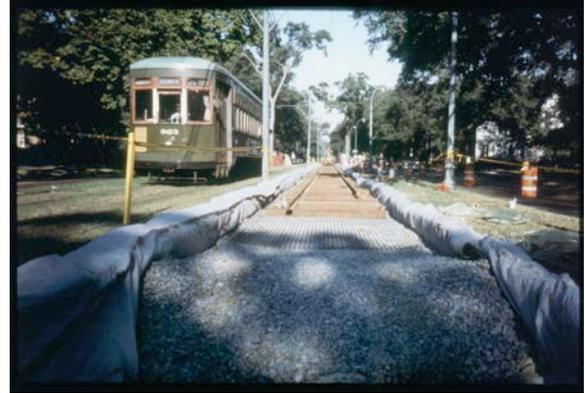
This rail line reconstruction benefited from both a nonwoven geotextile and a reinforcing geogrid
