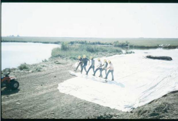
Large factory-fabricated panels are deployed on the jobsite.
