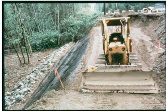
An RSS is constructed using conventional equipment.
