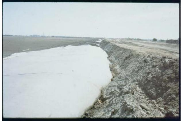
As the backfill is placed, the soft foundation soils begin to "mud wave".
