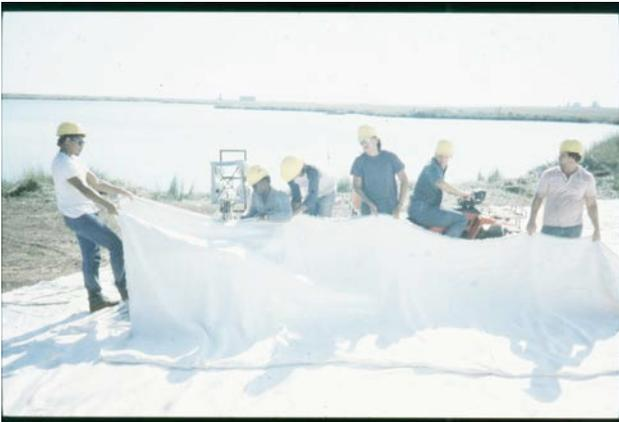
Factory-fabricated panels must still be field sewn into continuous sheets of reinforcement.
