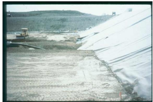
Clay (and then a geomembrane) is placed over a leak
