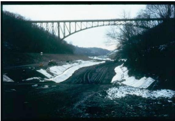
A geotextile sandwiched aggregate blanket drain protects this highway fill
