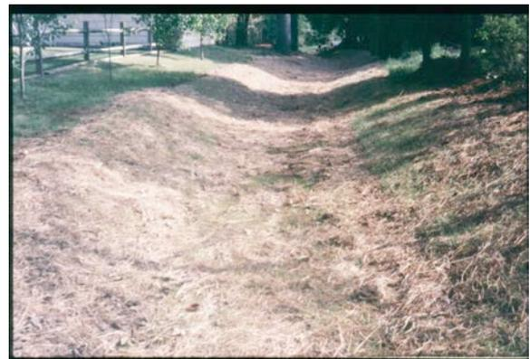
Channel installation includes: fine grading and seeding; RECP deployment and pinning; and backfilling and compacting. The resulting channel provides all the benefits of vegetation.
