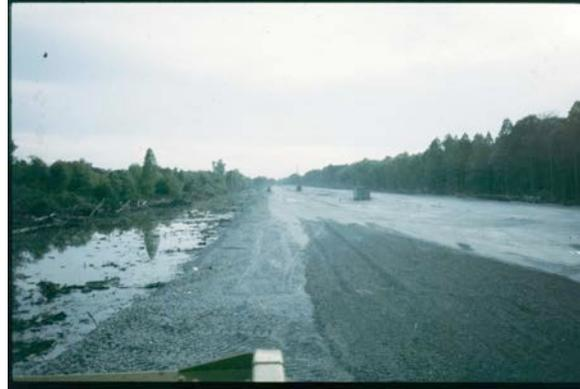
Stabilization geotextiles can be fabricated into large panels and deployed to expedite road embankment construction
