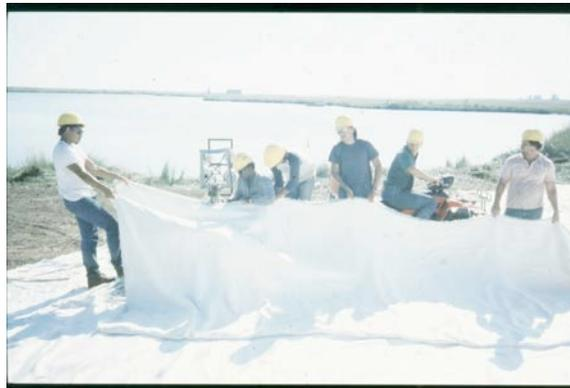
High Strength Geotextile Seaming
