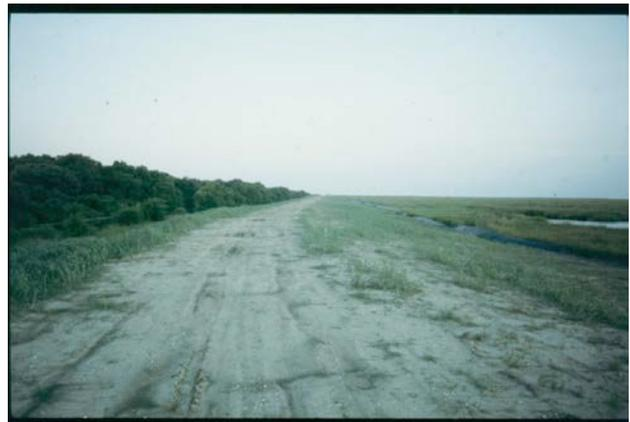
The completed embankment is taller and has steeper side slopes than would be possible without reinforcement or alternative stabilization.
