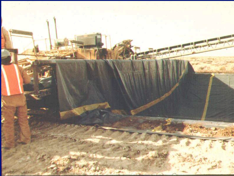
(Lining a Canal: Before Soil Covering)
