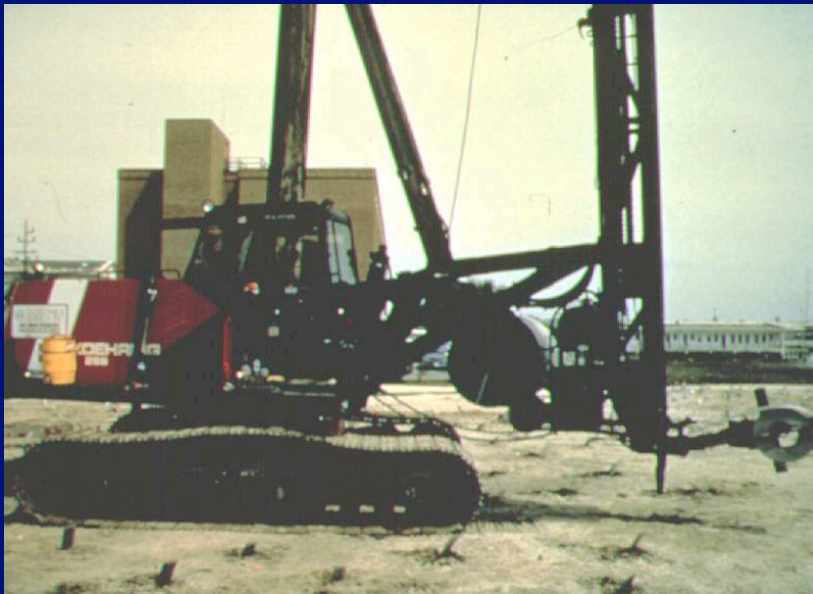
(Driving Wick Drains)
