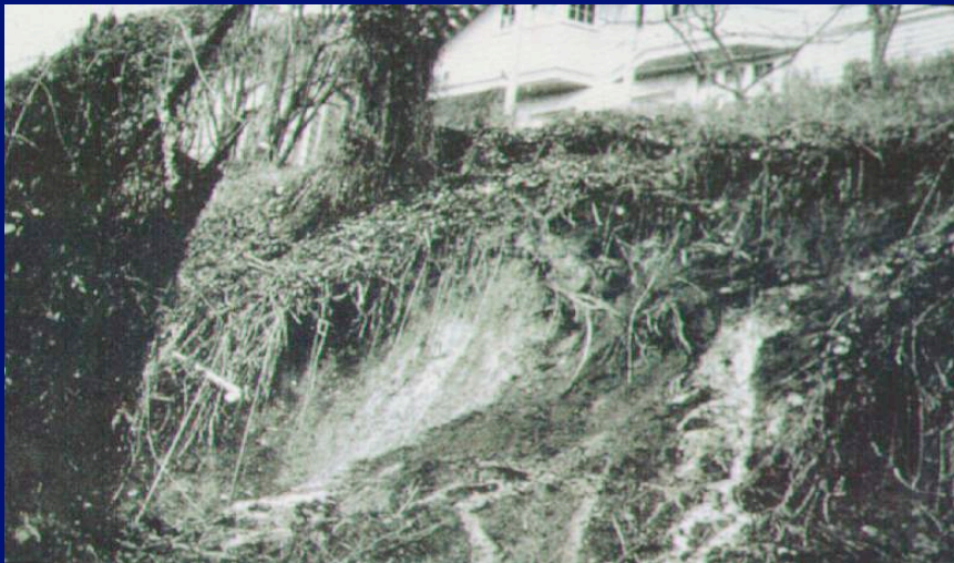
(One that Failed)!
