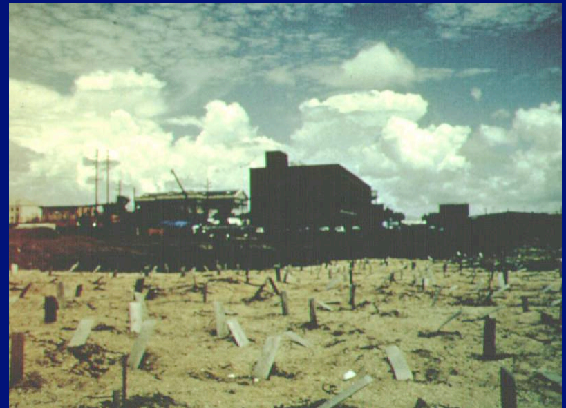
(Ready for Surcharge Fill)
