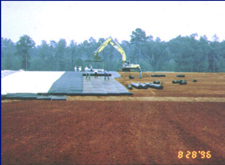
(Sequential Placement of GSs)
