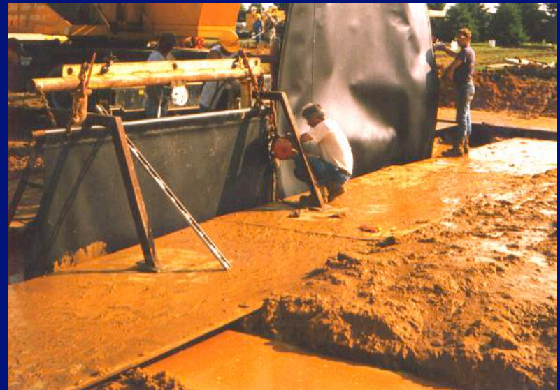
(Placement of GM Panels)
