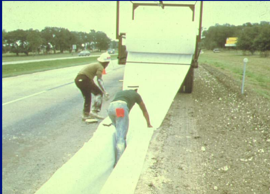
(GT Filter in Excavated Trench)
