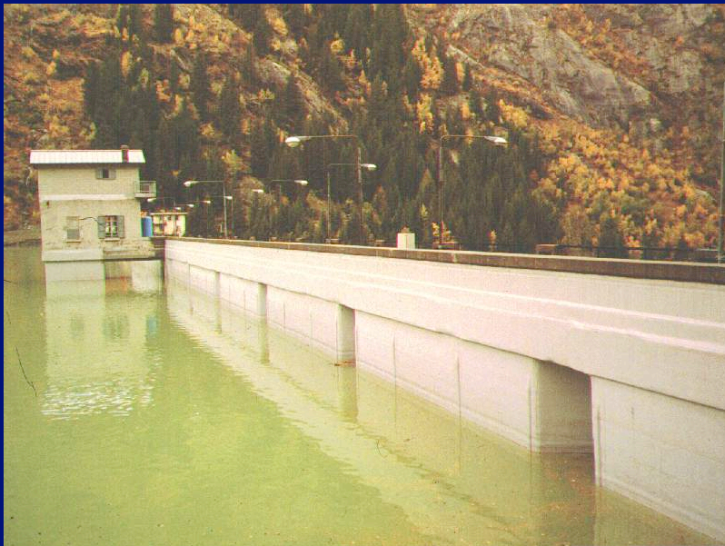
(Completed Concrete Dam Lining)
