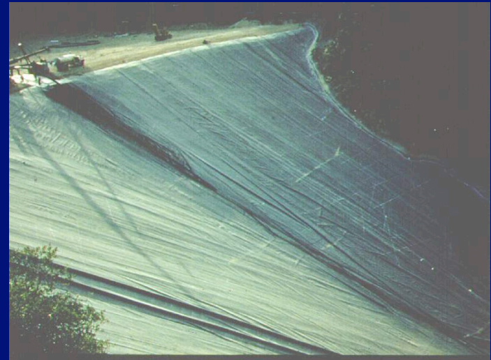
(Lined Earth Dam: Before Rip-Rap)
