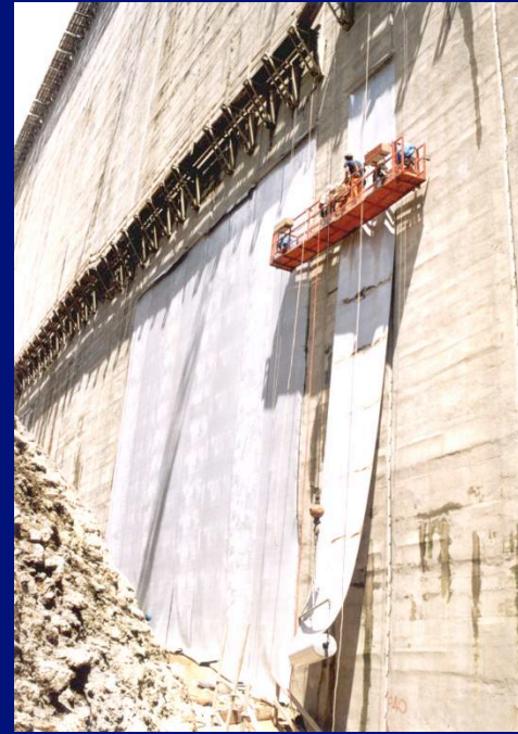
(Lining a Concrete Dam)
