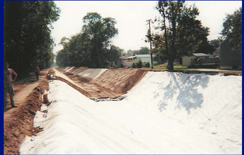
(GCL Lining of a Canal)
