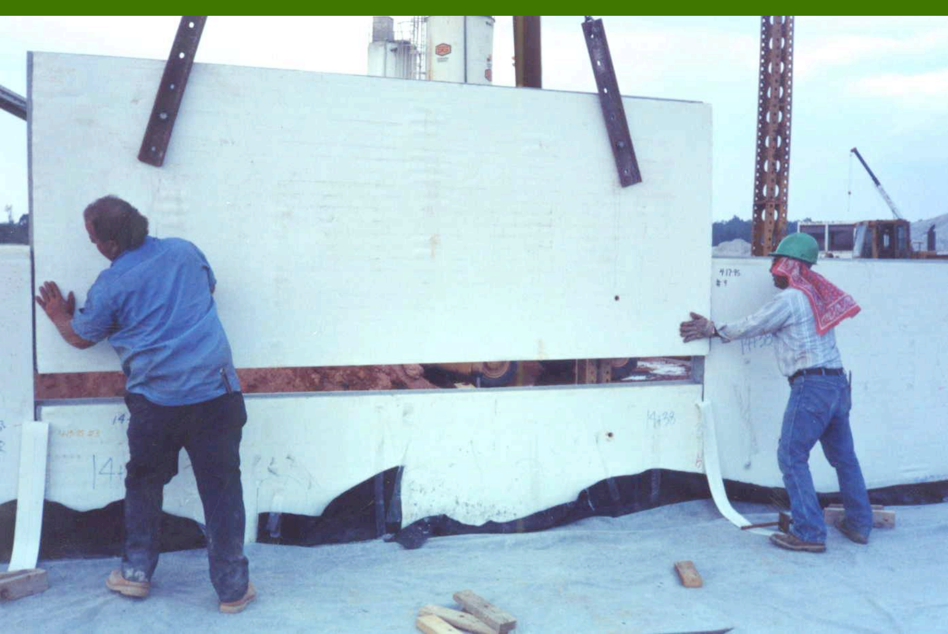
Cured Panels Being Placed; Note Edge Strips
