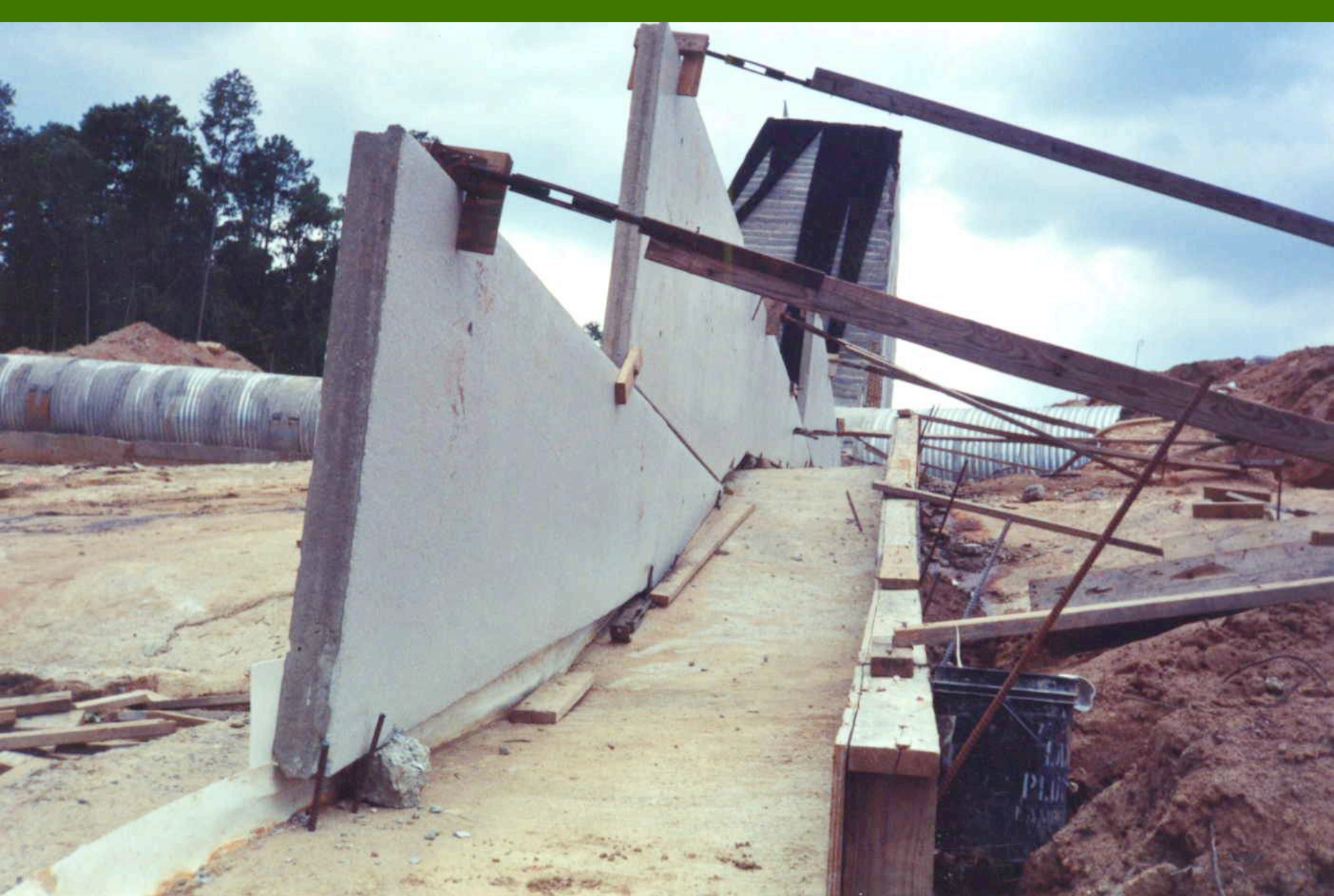
Initially Placed Panels; GM to Interior
