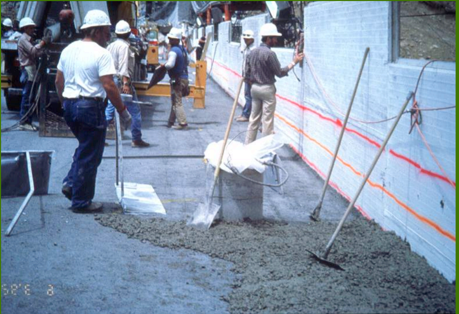
Placement of RCC Using Panels as Falsework
