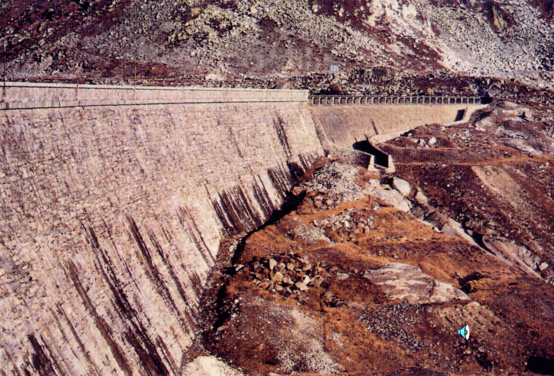
Downstream Masonry Dam Water Markings
