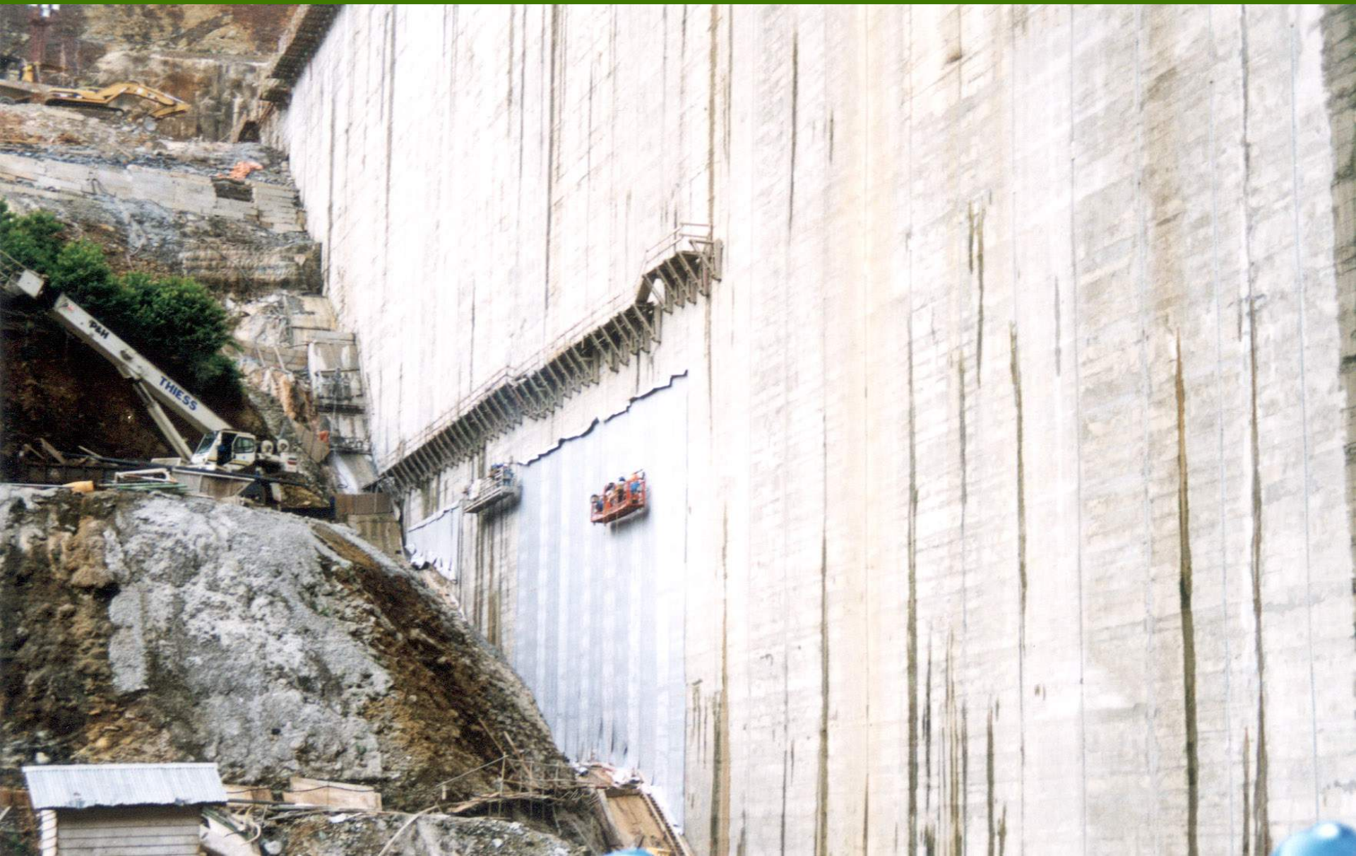
Work in Progress – Inserting Anchor Belts
