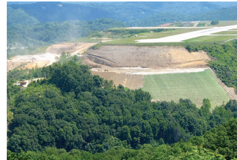
Construction in progress of a 242-ft-high geogrid reinforced slope. The completed slope allowed for a 500 ft extension of a runway at Yeager Airport in Charleston, West Virginia.
